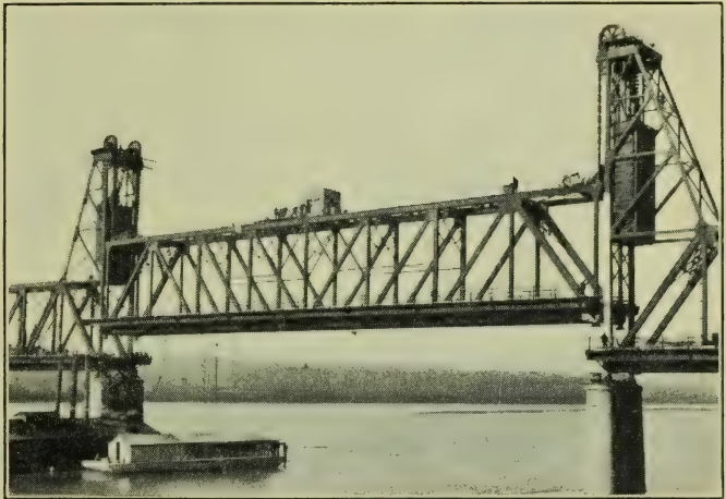
FIG. 10.—Vertical Lift Bridge Over the Arkansas River
